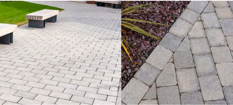
3 - Precast block paving to shared amenity space
