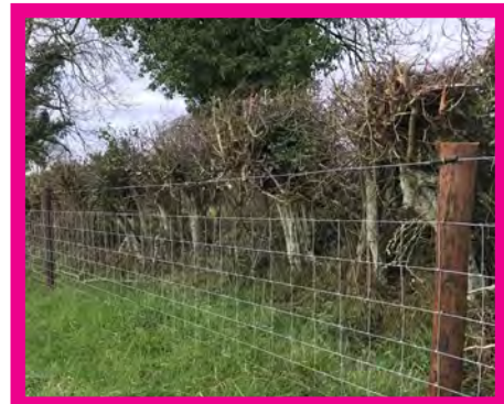
FFG02 - 1.2m High Post and Wire Fence to Garrynafela Stream
